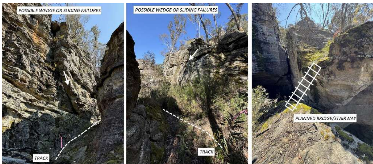
Figure 3-5: Trackside photographs of rockfall hazards in Section 2 above unnamed creek crossing
