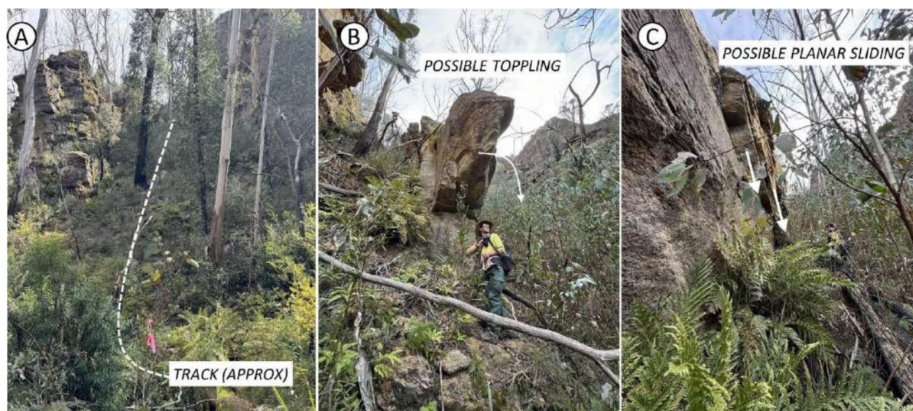
Figure 3-3: Trackside photographs of rockfall hazards in Section 1 above Carne Creek crossing
